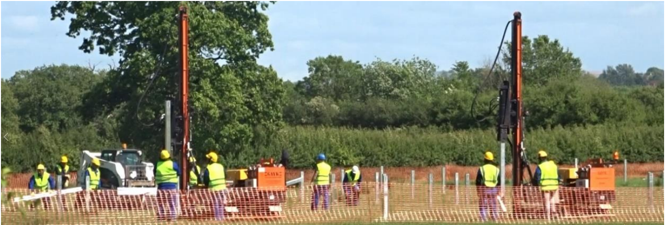
Plate 15.142: Legs being Installed
