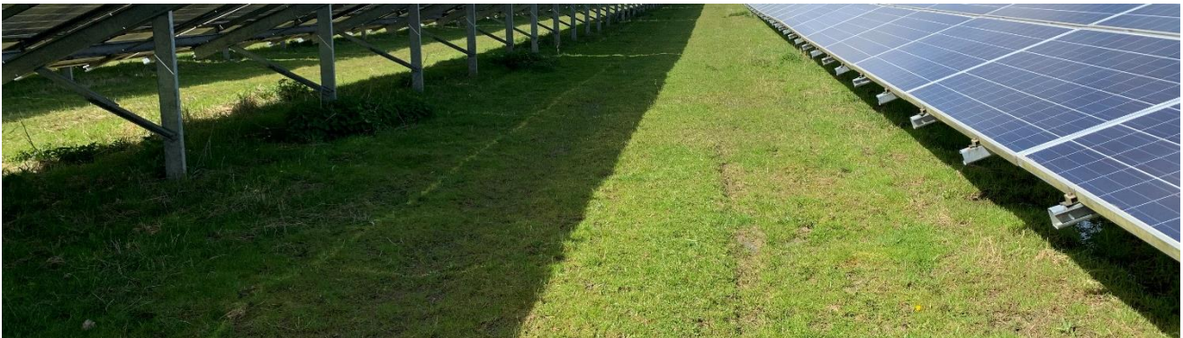
Plate 15.1920: Example of Minor Rutting by Maintenance Machinery
